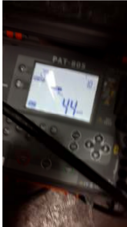
Photo 15 - The test cabinet earth bond continuity test
